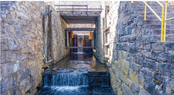
Historic Preservation of the Canal Lock
