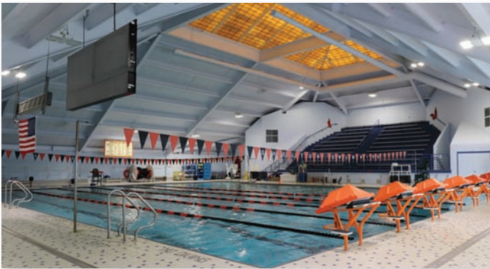
Community Center Pool
