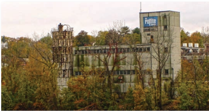
Rolfite Demolition / Remediation
