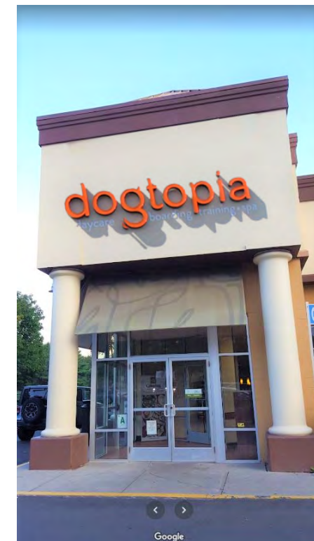
FRONT ENTRANCE MOCK UP
