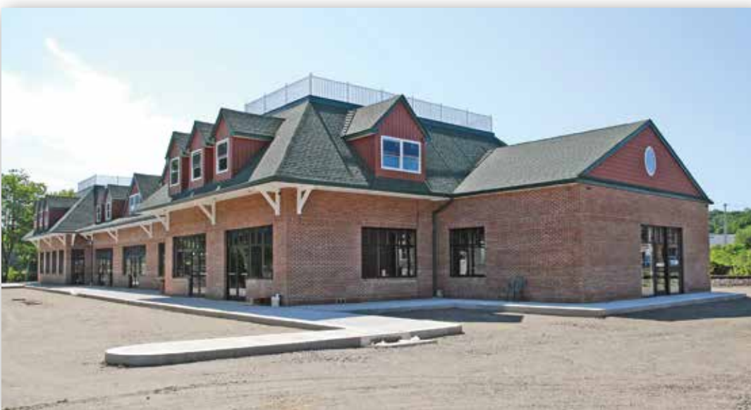
The once contaminated Rolfite site is now the home of new commercial construction.
