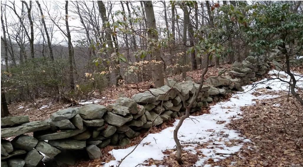
Photo: A long stone wall runs along the top of the steep slope, parallel with Mill Street.
