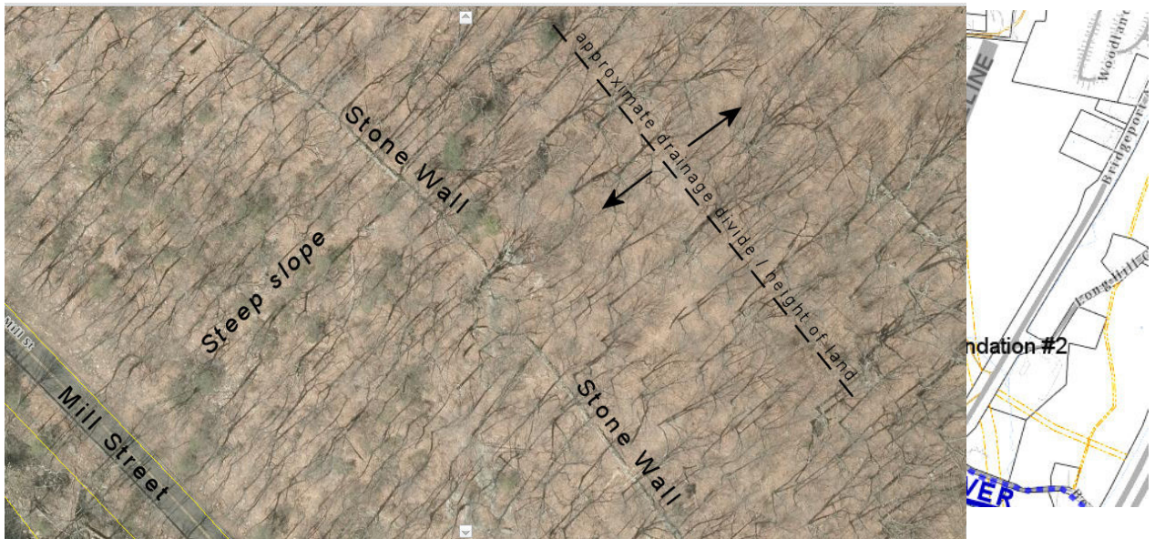
Aerial showing a portion of the long stone wall at the top of the steep slope along Mill Street.
